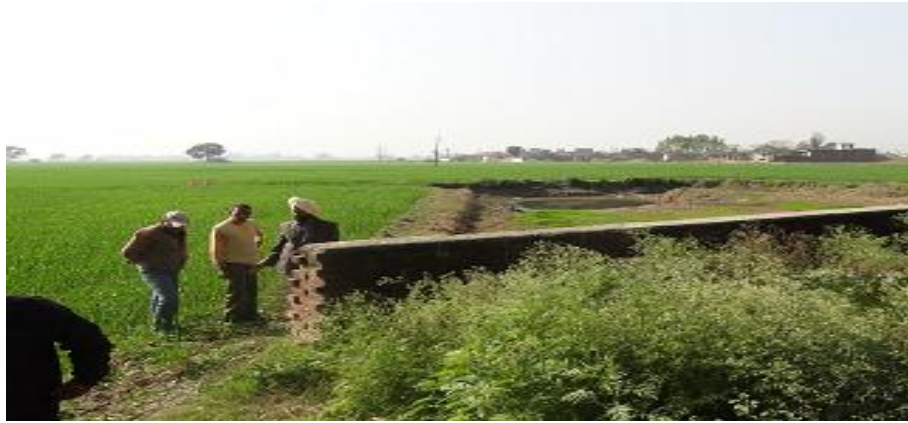
Desilting & Retaining wall of pond, Village: Miani Jhabelan Block: Dinanagar
