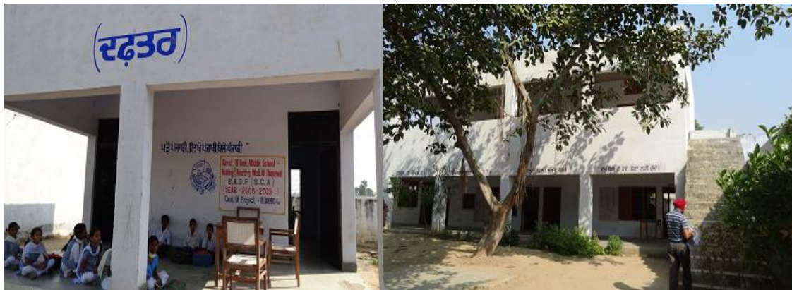
Room of Govt. Middle School, Thanewal
