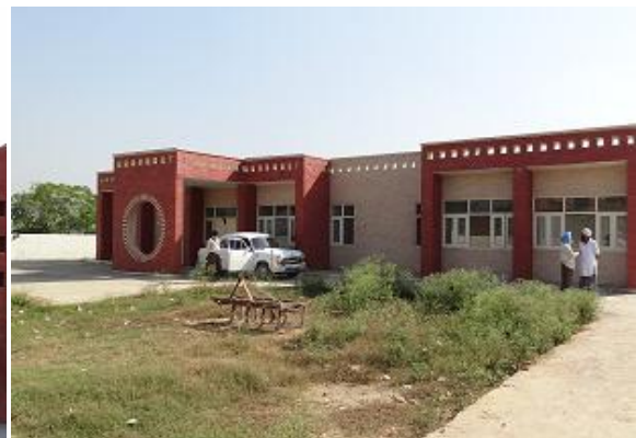
Construction of Mini Public Health Centre Building, Village: Dalam , Block: Dera Baba Nanak
