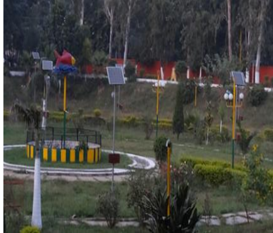
Installation of solar light in Fish Park, Gurdaspur
