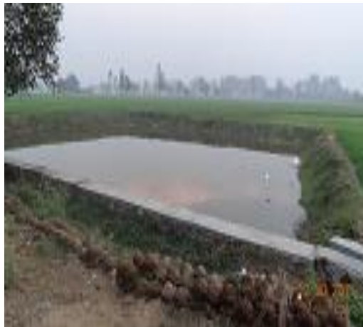
Desilting/Excavation of village Pond - Chak Amir, Block Bamial
