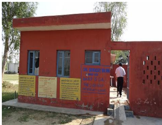
Construction of Civil Dispensary Building, Village: Talwandi Virk Block Gurdaspur
