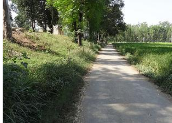
Construction of link Road in area of BOP Metla under 49 Bn. Village: Metla Block: Dera Baba Nanak
